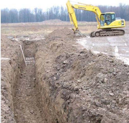
Figure 7. Excavating for the horizontal geothermal loop field. A horizontal installation was selected as a more affordable alternative to a vertical loop field.
